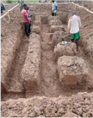
New toilet block under construction.
